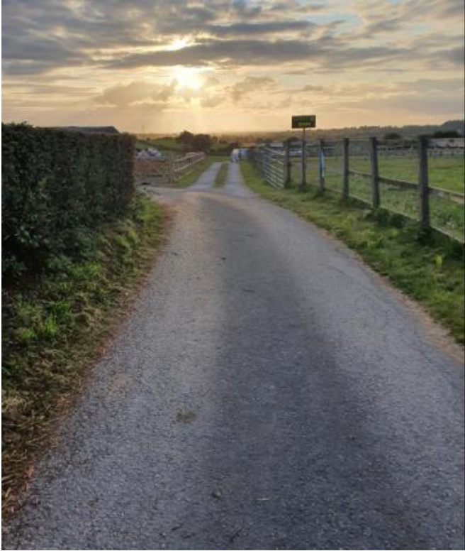
Figure 1: Blind Bend No 1 leading into our property from Stoney Low Lane.
