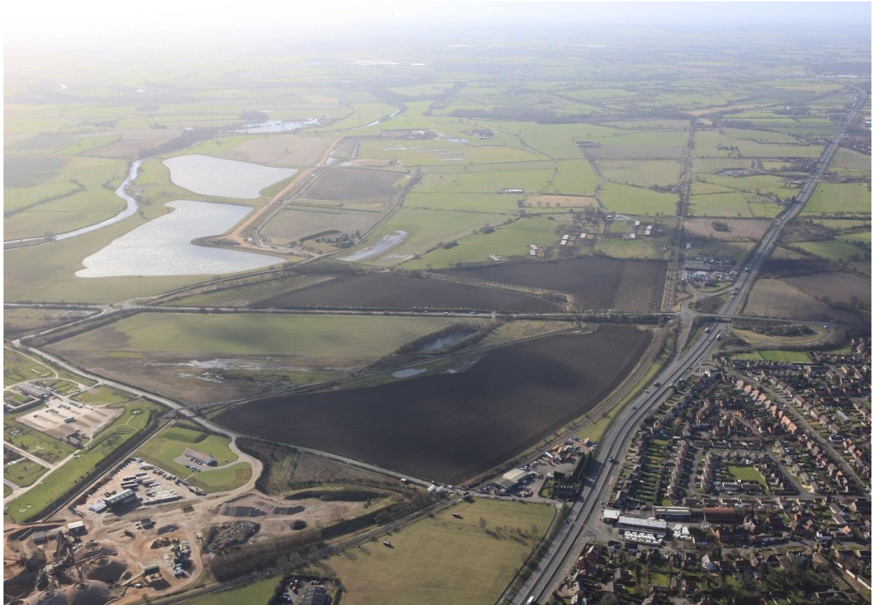
Figure 1: View of allocated site extension, looking southwards with plant site and National Memorial Arboretum (bottom left) – Alrewas village and A38 (right hand side of photo) – restored Whitemoor Haye area with lakes (top left) [c.2008]
